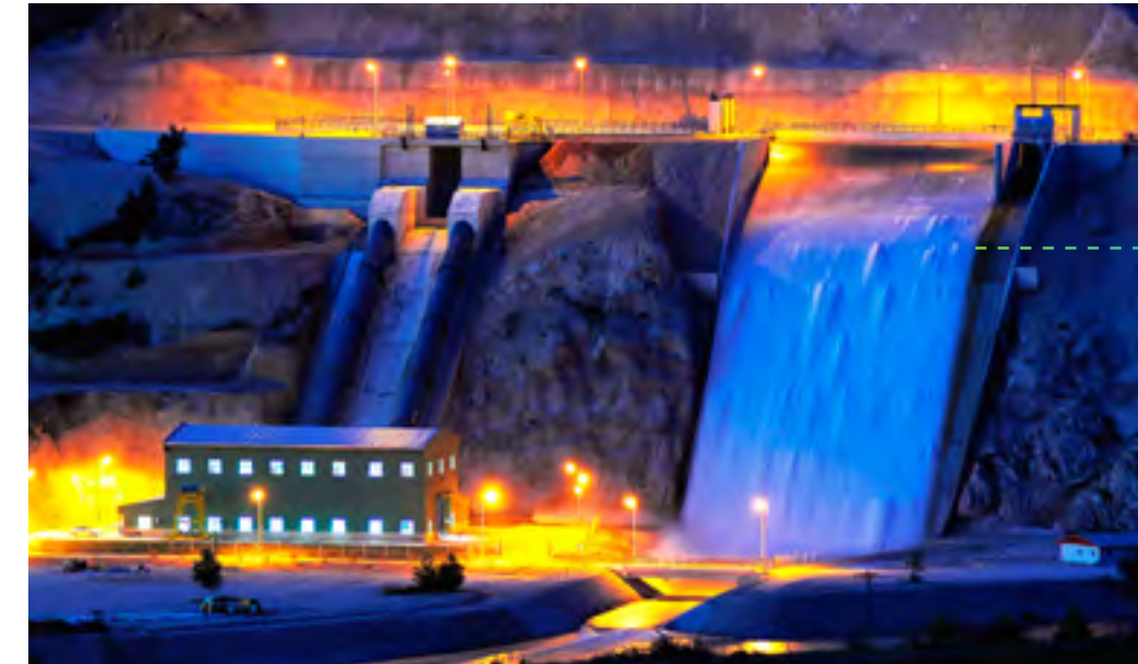
Niksar Hydroelectric Power Plant
