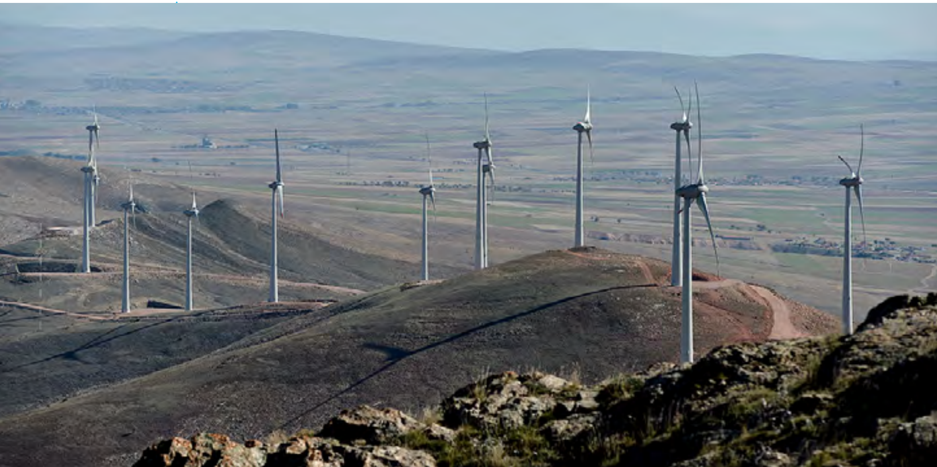
Geycek Wind Farm
